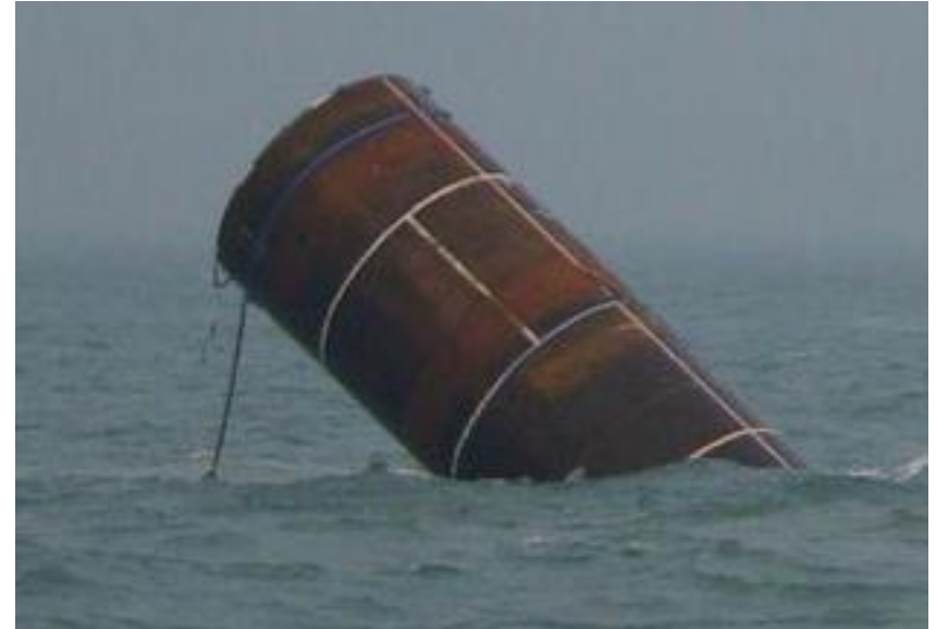
A monopile sank and was damaged
