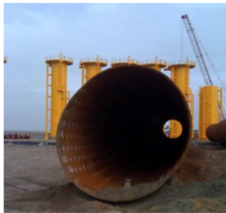
An « oval » foundation after it sank during transport to site
